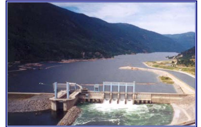
The Keenleyside Dam on the Columbia River near Castlegar B.C.
